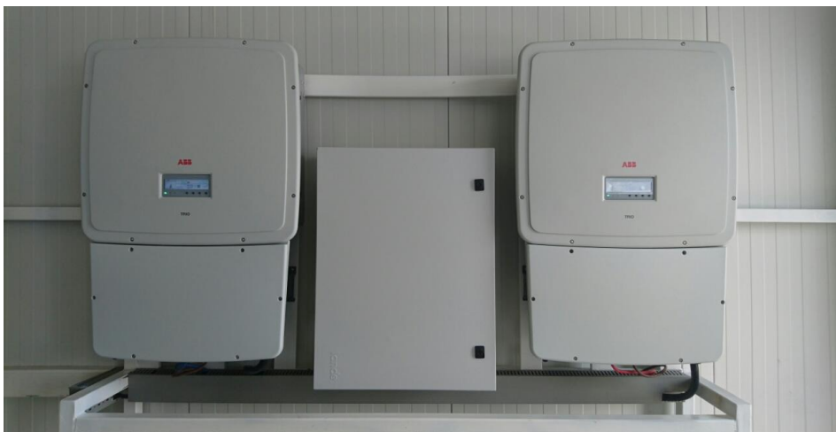
Fig. 8.3 Inverteret ABB TRIO-27.6-TL-OUTD-S2 -400
