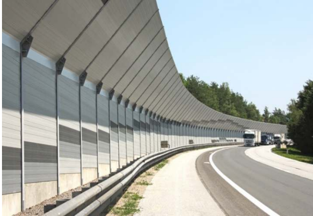
Fig 4.19 Barriera metalike (celik apo alumin) [25]
